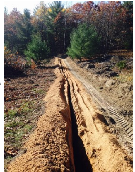
Trench line for breaking root grafts at a parcel in Manistee County. Photo by Chad Van-Voorst.
